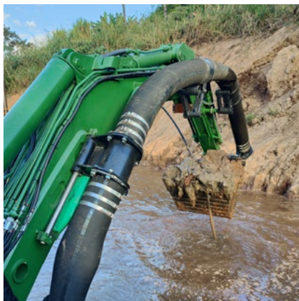
Watermaster excavating to open access for the other dredgers
