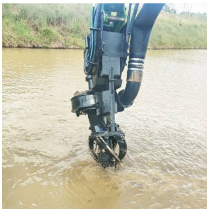
Watermaster dredging tailings with its submersible cutter pump (up to 900 m 3 /h)
