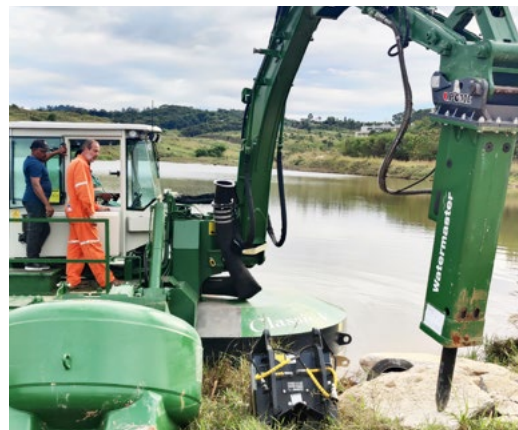
Stones in the river can block access. Watermaster breaks them with its hydraulic hammer to open the way
