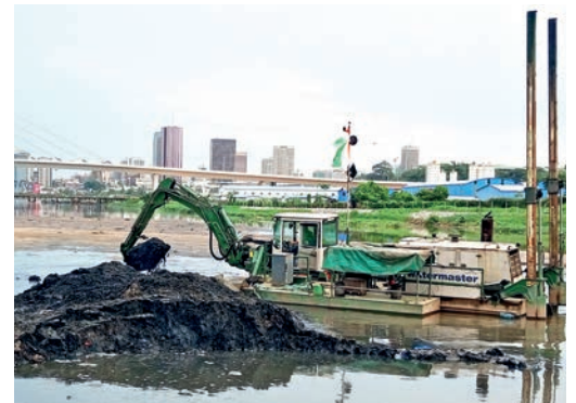
Canal maintenance work in the Ivory Coast
