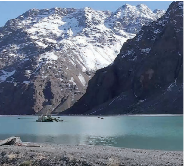
LINED RESERVOIRS FOR INDUSTRIAL USE
