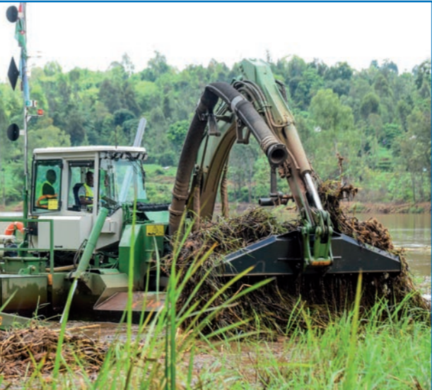
REMOVE EXCESSIVE VEGETATION BY RAKING
