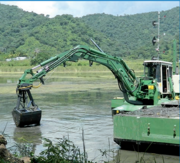
CLEAR SEDIMENT AND REEDS BY EXCAVATING
