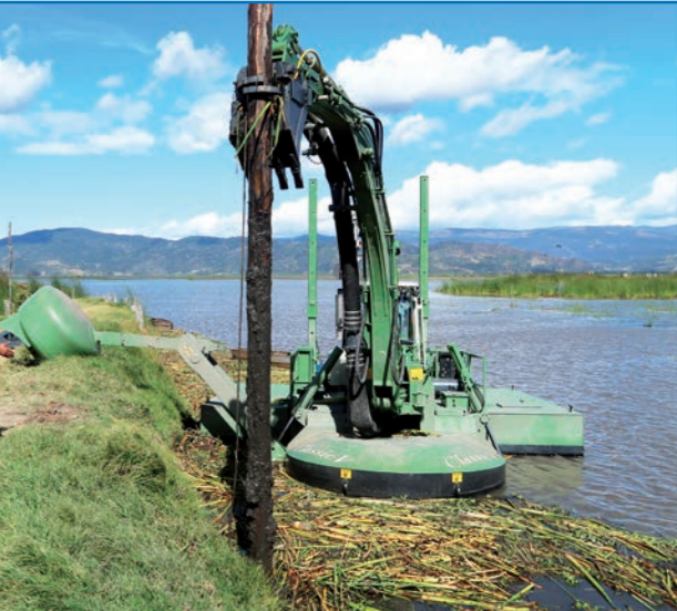
STOP SHORE EROSION BY PILE DRIVING
