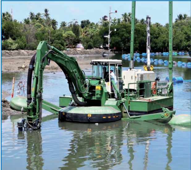
DESILT BY SUCTION DREDGING
