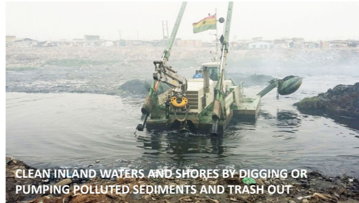
MAINTAIN THE NAVIGABILITY OF WATERWAYS AND PREVENT FLOODS BY DREDGING AWAY EXCESS SILTATION
