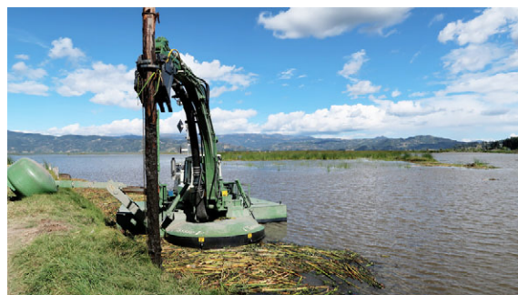
Pile driving work at Lake Fúquene
