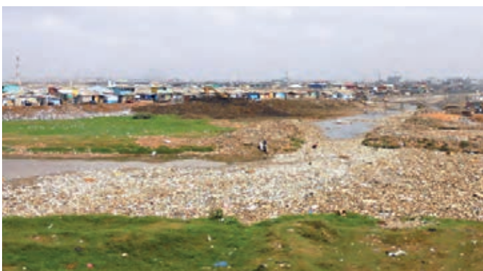
Pollution, excessive siltation, poor water flow, high risk for floods
