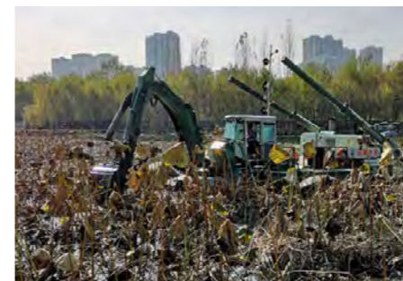
Removing waste and siltation by excavating
