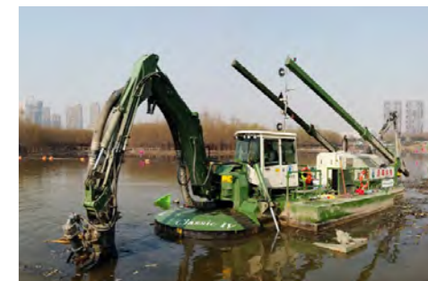
Removing sludge by suction dredging
