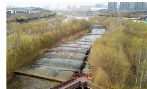
Dewatering with geotextile tubes
