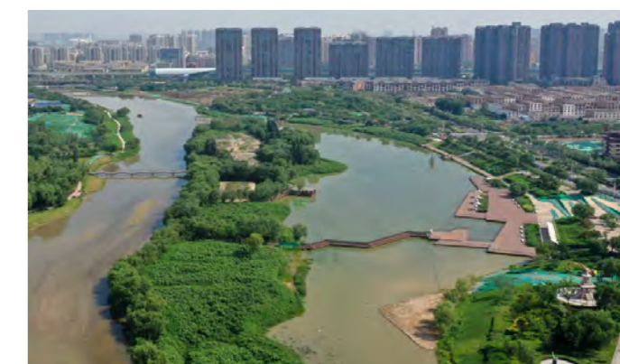
AFTER restoration Cleaner and healthier environment and recovering ecosystems, more enjoyable urban area for locals and tourists, lower risk of floods
