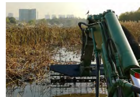
Clearing vegetation and debris by raking
