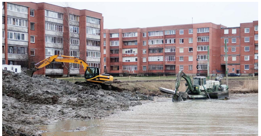
Desilting work - Silt and sediments accumulate in the bottom of rivers and canals over time. Desilting these deposits reduces flood risk and improves water flow (picture from Lithuania)
