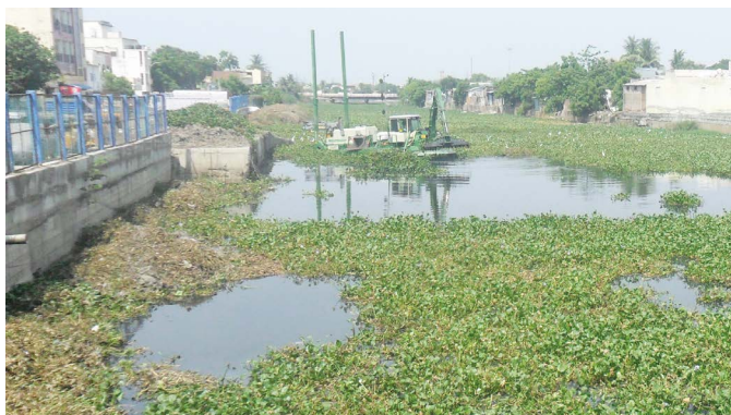
Invasive water hyacinth and excessive silt cause many problems
