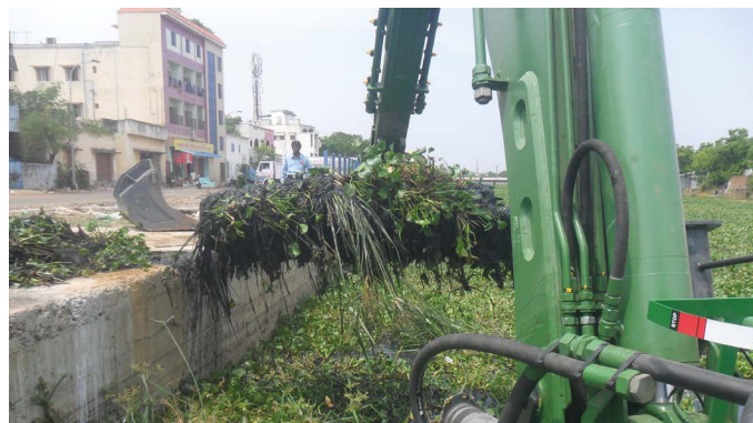
Watermaster raking the silt and vegetation out of the canal
